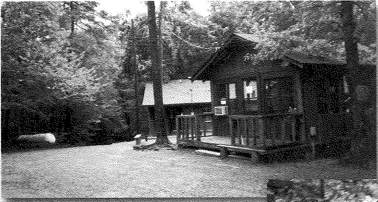
Office Bath House Below
